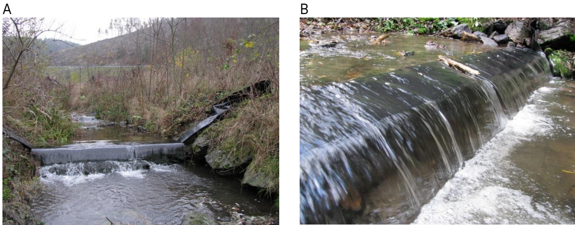
Fig. 1. Temporary migration barriers at Besének stream: A) modified masonry/concrete step, B) detail of a modified overflow edge on a log step.
