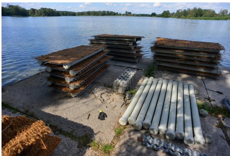
Fig. 1. Gabion-based construction of floating artificial islands (photo: Tomáš Jůnek)
