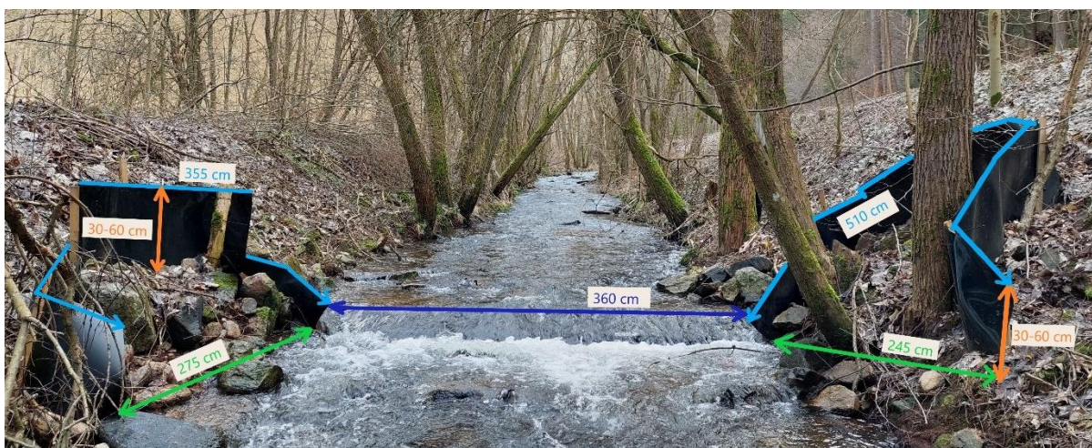
Fig. 2. Design and dimensions of the modified step on the Besének stream. Experimental verification of the passability for the signal crayfish was carried out on these steps (Image by B. Šrytrová).
