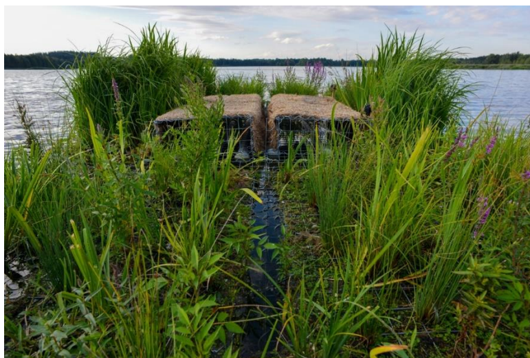
Fig. 2. Plants secured with coconut material, Krvavý fishpond (photo: Tomáš Jůnek)
